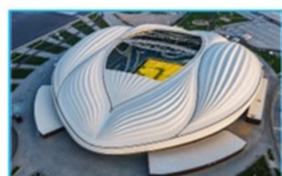
Al Janoub Stadium - 40,000
