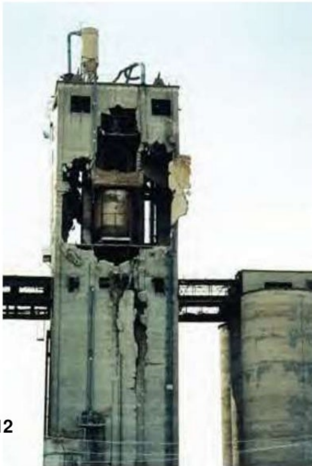
Damaged headworks of grain elevator.
